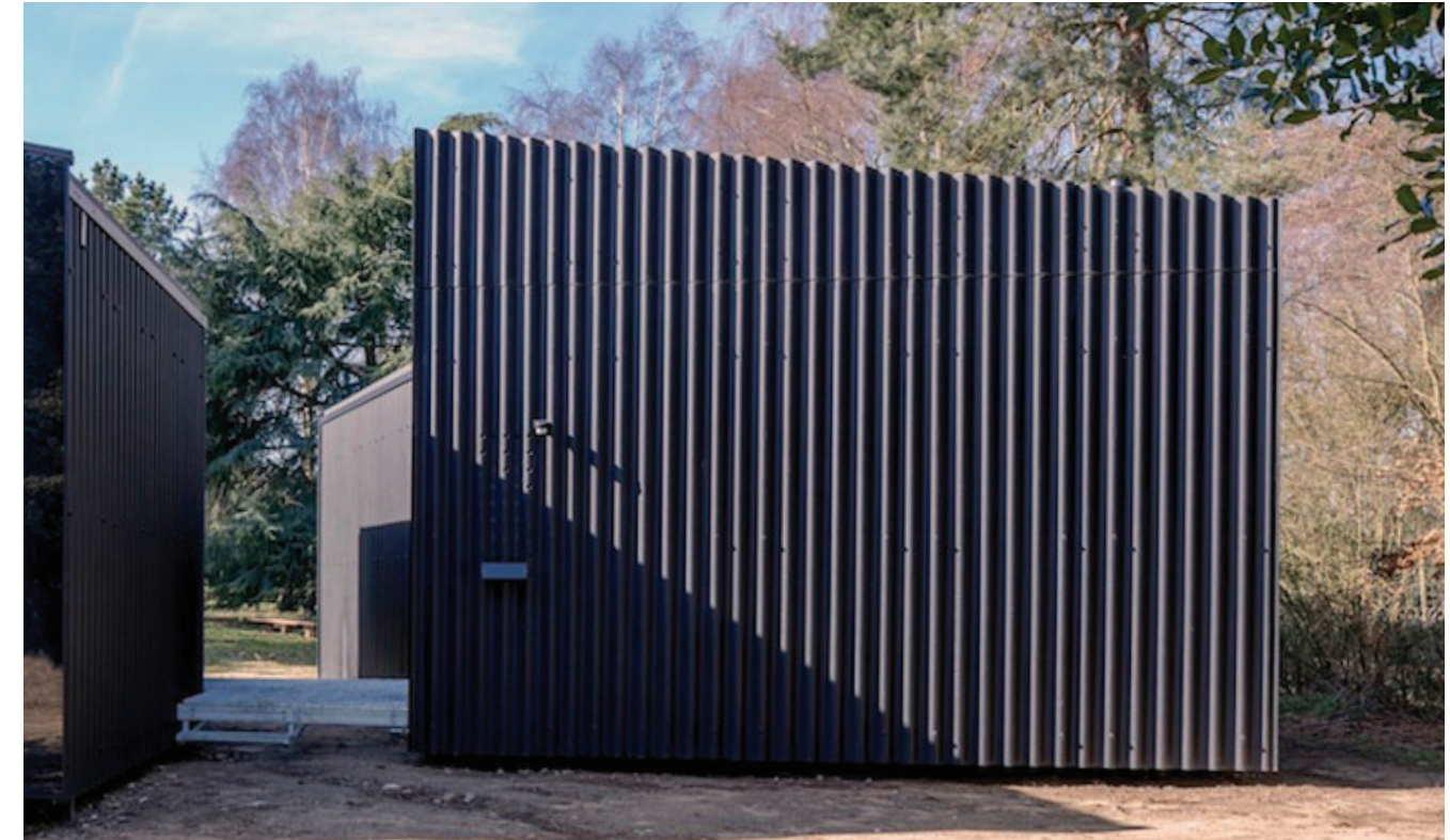
Figure 11: Fibre Cement Example 1
