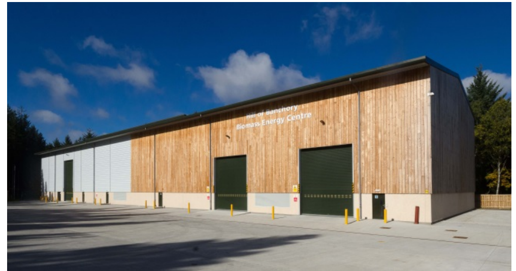
Figure 4 Biomass centre with wooden cladding
